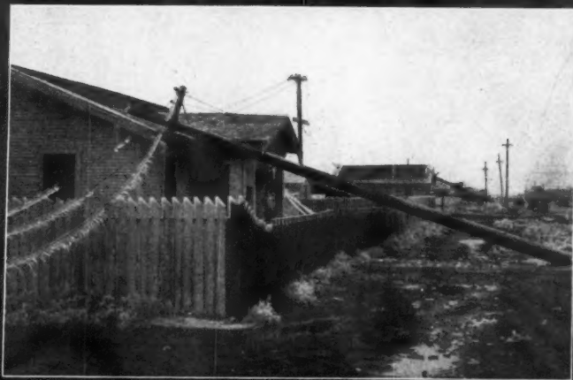
The severe ice storm which struck Amarillo, Texas, late in November left hardly a span of telephone or power lines undamaged. Upper left, a typical joint construction pole showing the tangled mess of wires left by the storm. Upper right, trees throughout the city suffered untold damage. Center, lines in the Santa Fe railroad yards. Below, other typical scenes.
